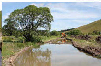
2013 July - cutting the new channel
