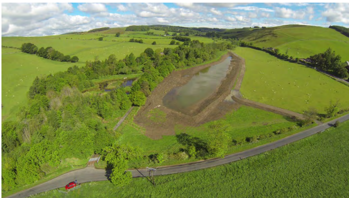
Aerial view of large flood storage pond at Kidston Mill – under construction
