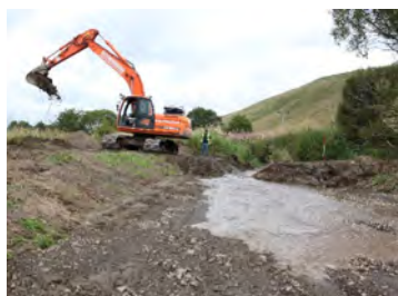
2013 August - Opening of new meander & first flow going down the channel
