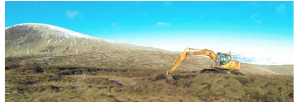
Digger in action at the Winterhope site, re-profiling extensive peat hags
